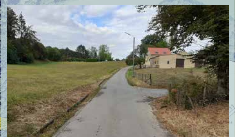
Station de pompage Wolpert
